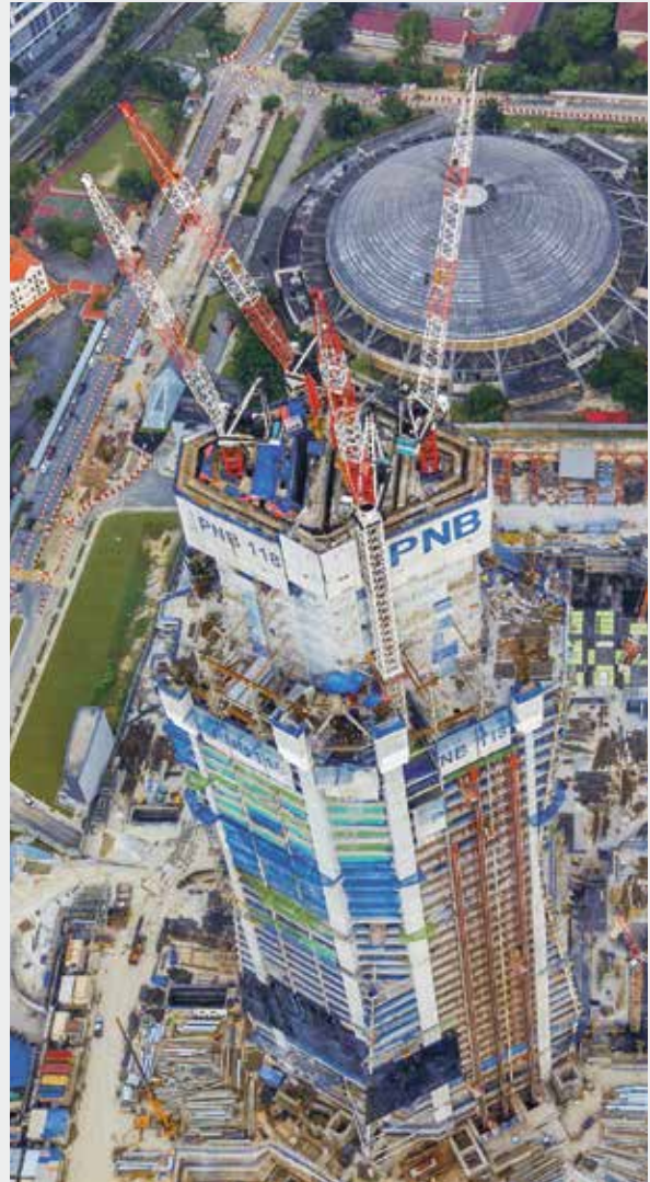
Tower crane, KL118, Malaysia
