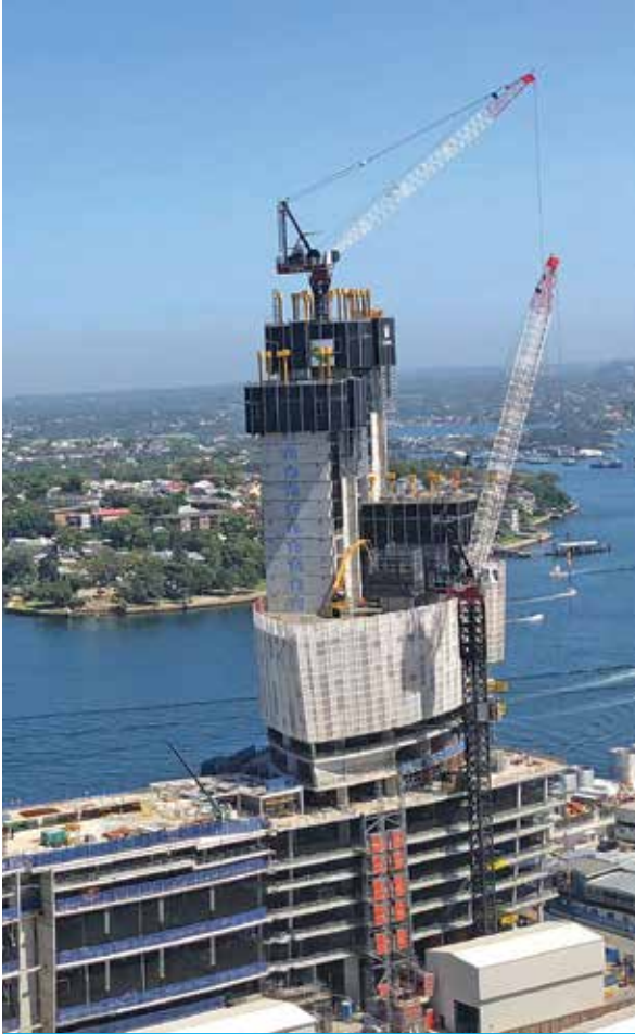
Tower and Offshore crane, Crown Sydney, Australia
