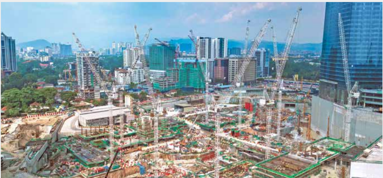
Tower crane, Tun Razak Exchange, Malaysia
