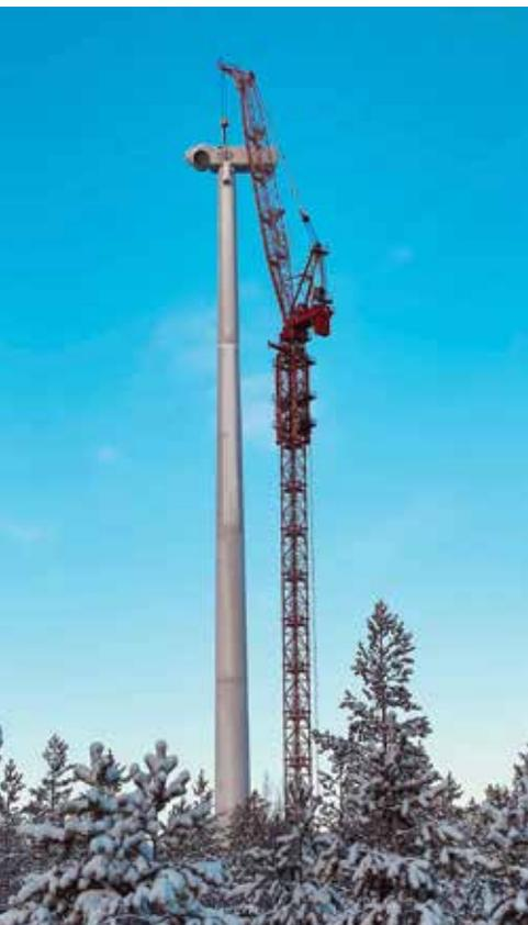
Tower Crane, Wind Turbine Column
