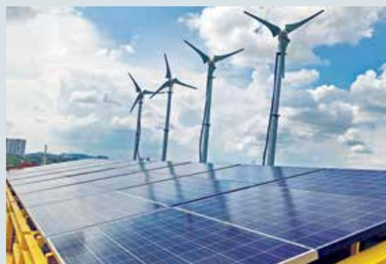
Solar Hybrid Wind Turbine System for Tembakai Non Associated Gas Wellhead Platform
