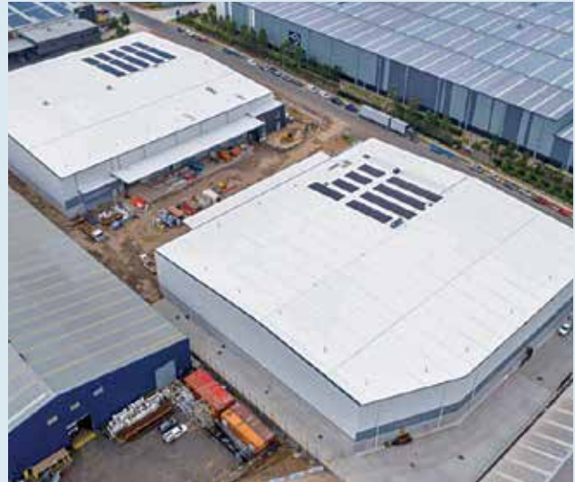
Two units Single Storey Warehouses in Sydney, Australia
