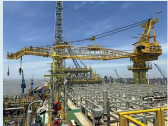
Offshore Crane, Yinson Bergenia Production B.V., China
