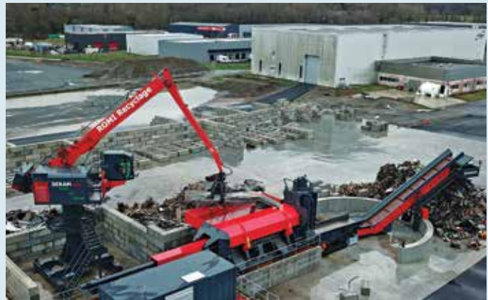
Equilibrium Crane installed at Artois Métaux, France
