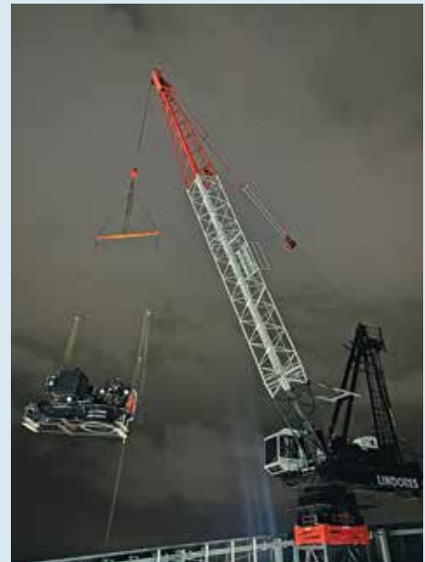
Tower Crane Recovery Process, Lindores Construction Logistics, Australia
