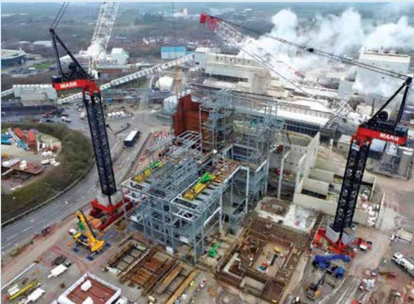
Tower Crane, Lostock Sustainable Energy Plant, United Kingdom
